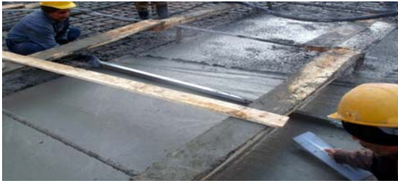
Fig. 9. Removing excess concrete and manual trowelling.
