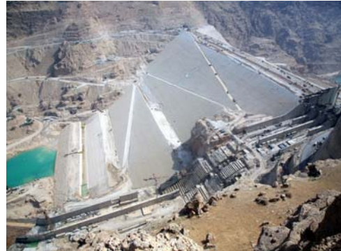
Fig. 1. General view of spillway structures, located on left abutment.
