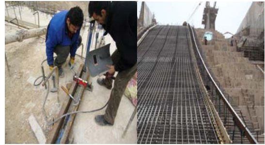
Fig. 15. U-Shaped beams and rail preparation.
