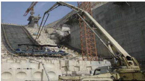
Fig. 17. Concrete transference by mobile pump.
