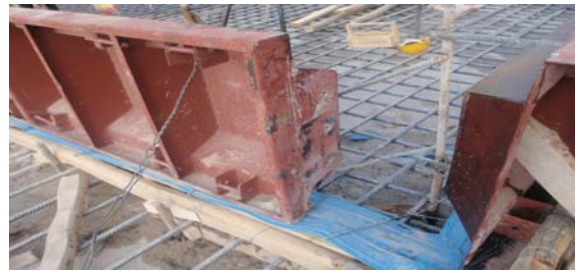
Fig. 12. Unusual metal formworks for apron block hydraulic faces.
