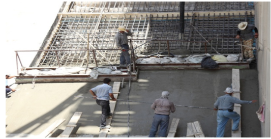
Fig. 4. Ogee concrete placement using scape form, DE part.
