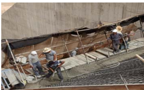
Fig. 19. Concrete placement underneath formwork.
