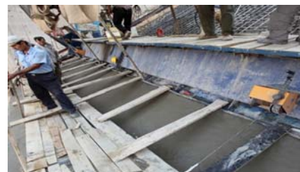
Fig. 22. Slip- Form forehead- connecting winches for workers plank.
