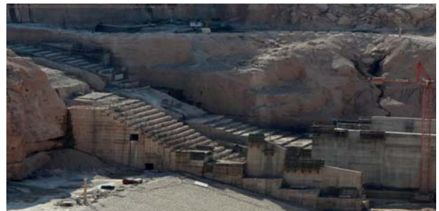
Fig. 13. Middle chute, underneath stair shaped mass concrete.
