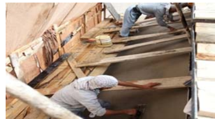
Fig. 21. Hanged platform and finishing operation by trowel.
