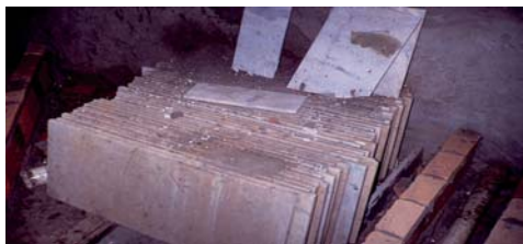
Fig. 9. Rocky material inadequate storage in construction site. may cause permanent staining before and or after placement.
