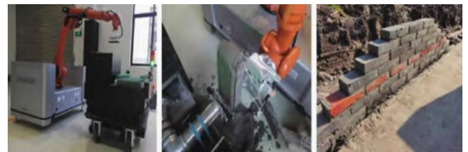
(a) Bricklaying Robot (b) Automatic Plastering Device (c) On-site Construction
